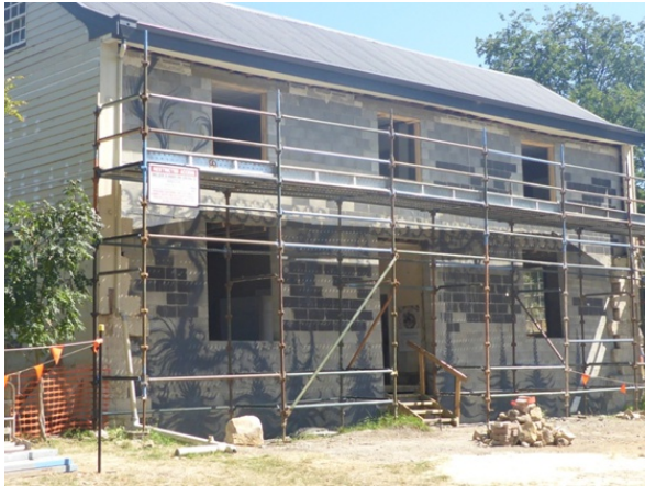
Patterdale Farm being restored
